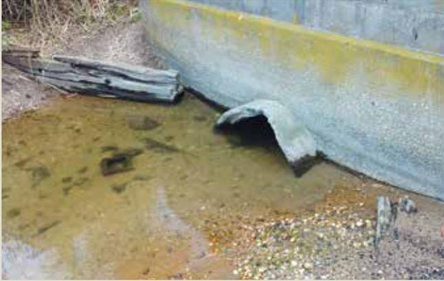
*Undersized and perched culverts limit connectivity and restrict fish passage*
