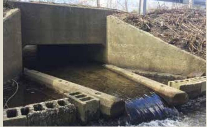
adult yellow eels. These devices are widely used in Europe and many off-the-shelf peg-board products are available. The 2016 modifications to the Peconic River dam at Edward's Avenue include a peg-board eel pass, the first on Long Island.
